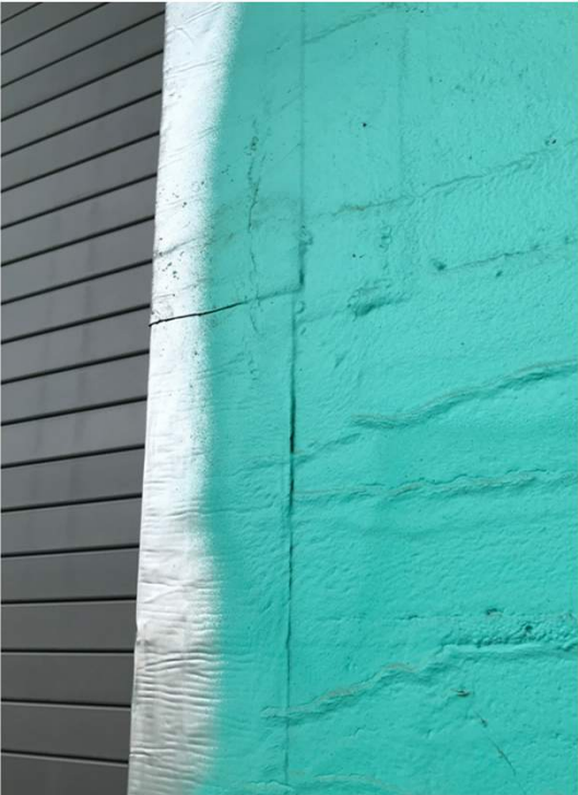
Low Adhesion – Asphaltic Products
