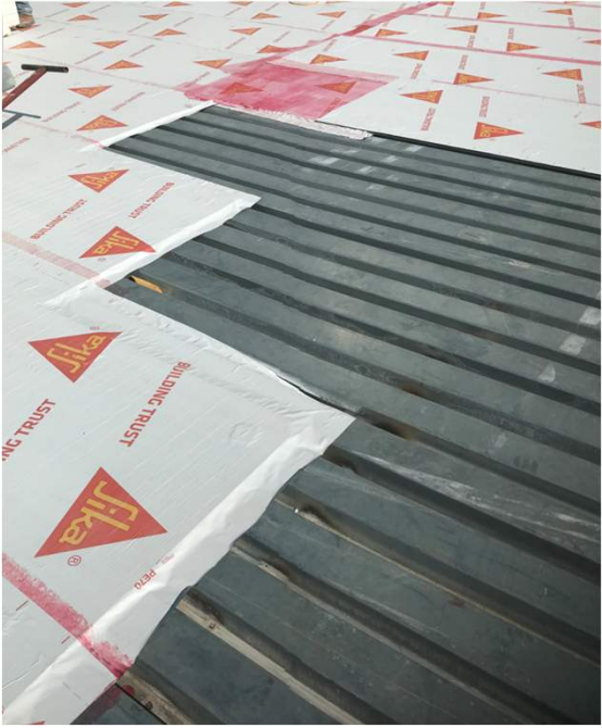
Roofing Night Seals
