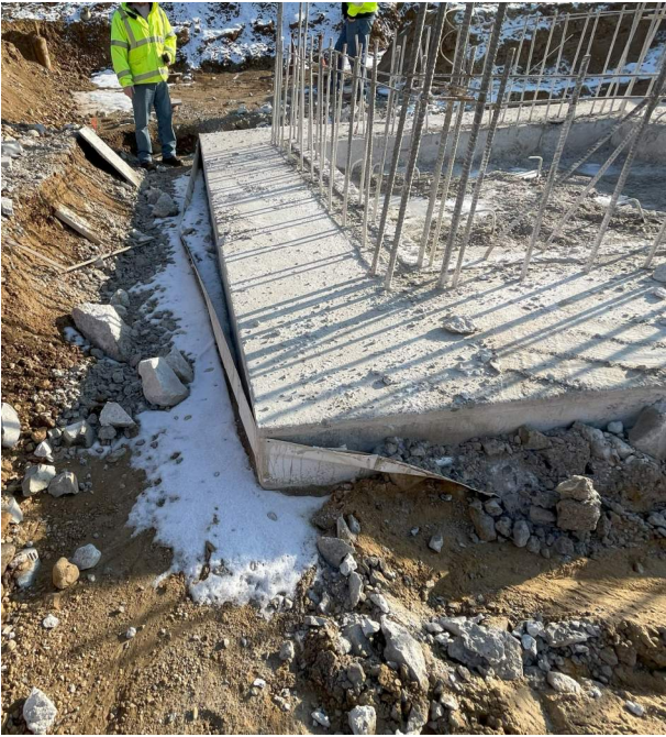
Waterproofing Damage
